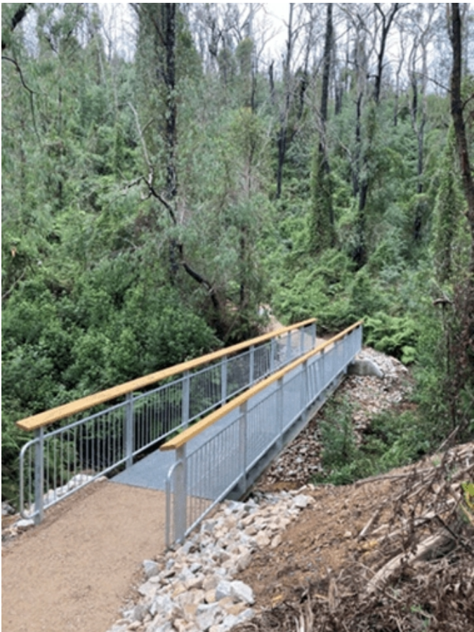
And the rebuilt bridge today, with regenerating forest. Credit: Parks Victoria
