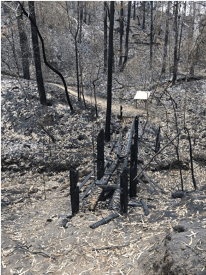
One of the Fairy Dell bridges in the aftermath of the Black Summer bushfires. Credit: Parks Victoria
